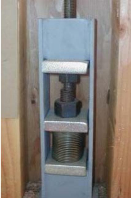
**h. Interfering Rod.** When cages are used rod cut length can be critical. If the rod is cut too long, the shrinkage compensator may expand and the rod ends can hit. Further expansion is impossible.
