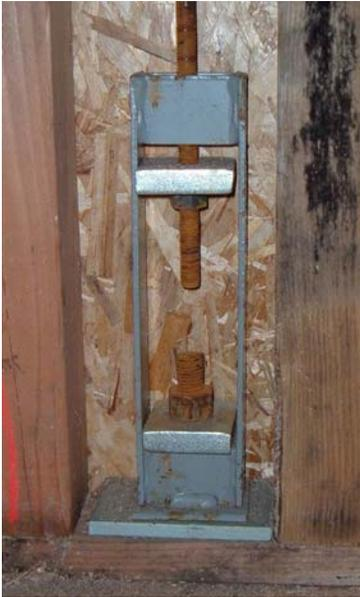
Jammed connections can be caused by: undersize holes, misaligned holes, pinched connectors, and out-of-square or out-of-plumb rod, out-of-square shrinkage compensators and insufficient headroom. With a jammed connection often the rod will buckle. Buckling is most common on the upper stories with lighter rod. Eight to ten feet of small diameter rod can easily buckle under the right conditions. If hidden behind sheet rock it may never be noticed.
