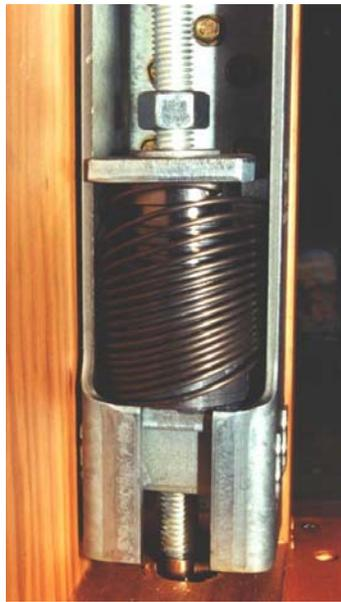
Some shrinkage compensators have external springs. As the devices expand vertically the springs expand horizontally. If the spring hits the side of the tie-down or enclosure the vertical expansion can be stopped.
